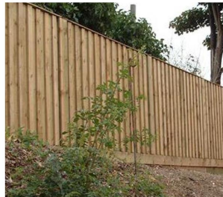
Img 28 - Timber acoustic fencing
